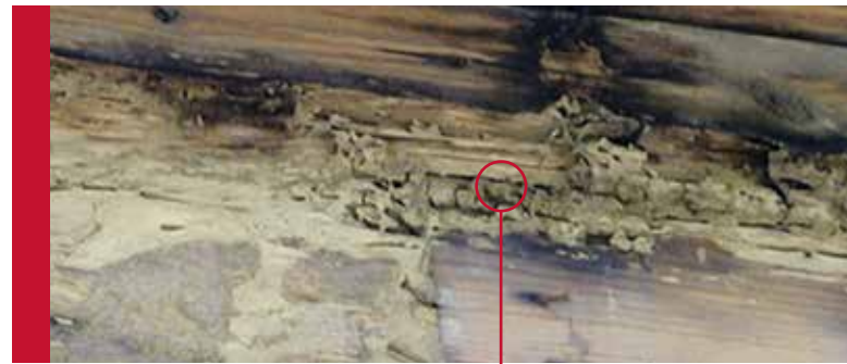
Termite Damage
